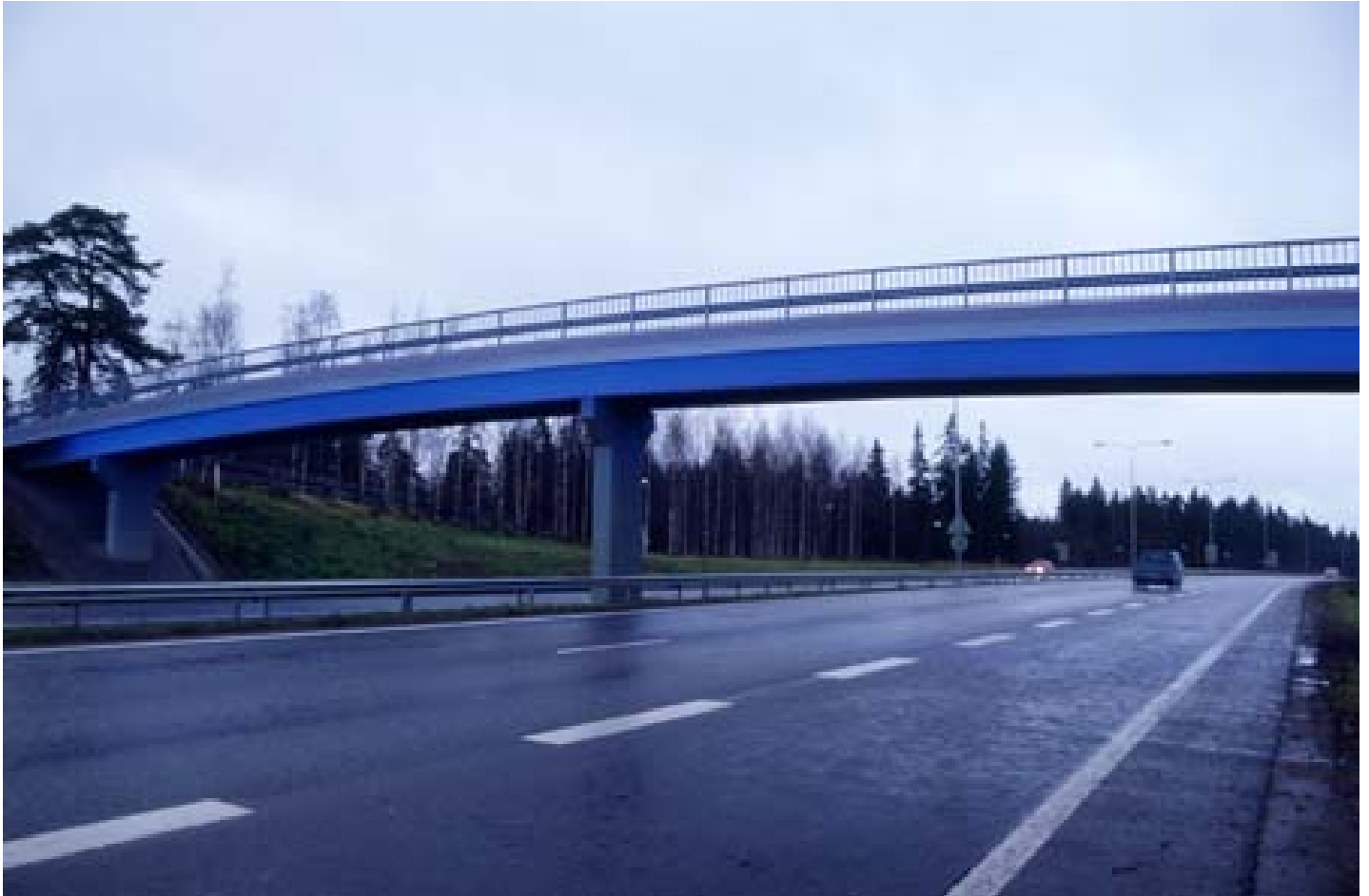
William Dennisuk, Speed of Light , 1997 lights, metal, paint, 100 feet, both sides Dennisuk,William.002
